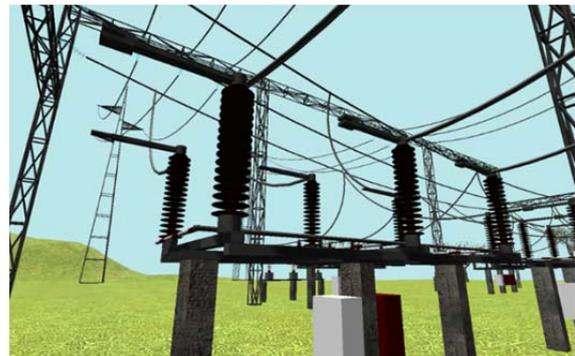
Figure 2. Open disconnecter 110 kV
