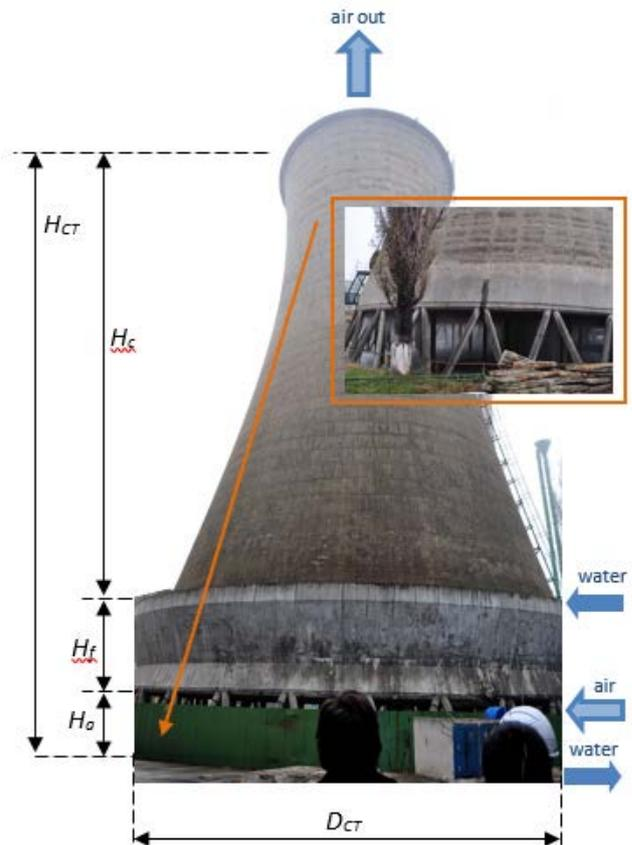
Figure 2. Counter-flow Natural Draft Wet Cooling Tower
